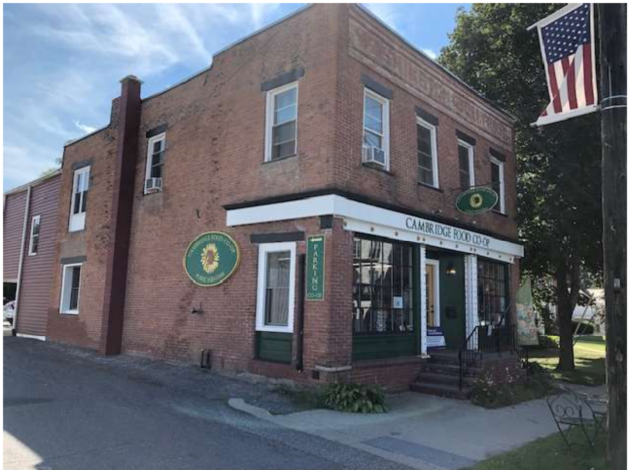
Front of Existing Building from East
