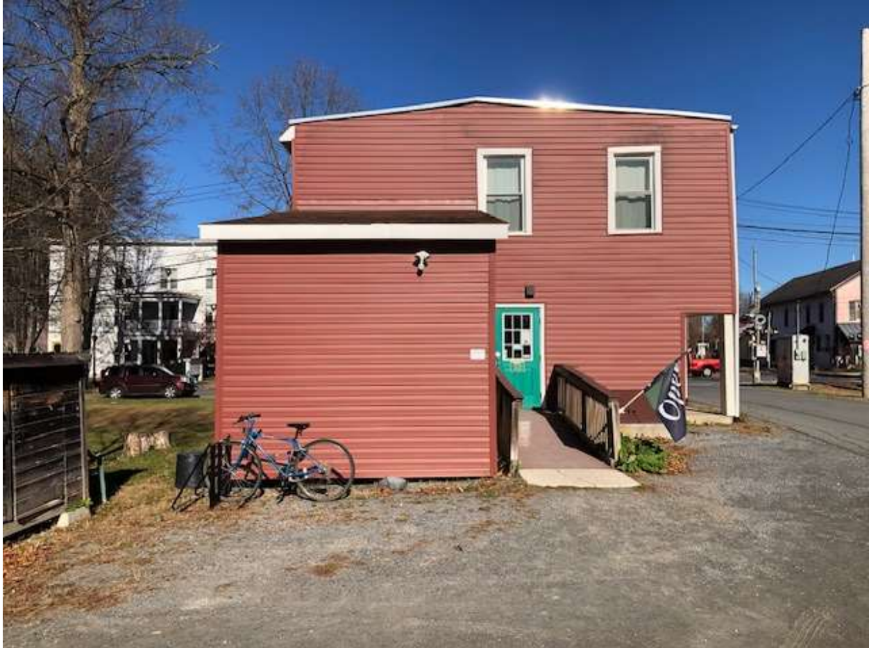
Rear of Building from South. Projection at the left is the enclosure for the current walk-in cooler which is to be removed. Proposed expansion will attach to this elevation.
